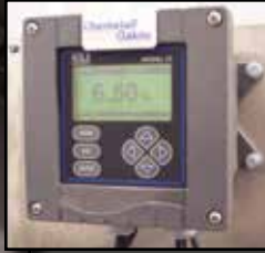
Automated Chemical Test Pretreatment chemicals are monitored and added automatically. Titration is checked manually twice per shift.
